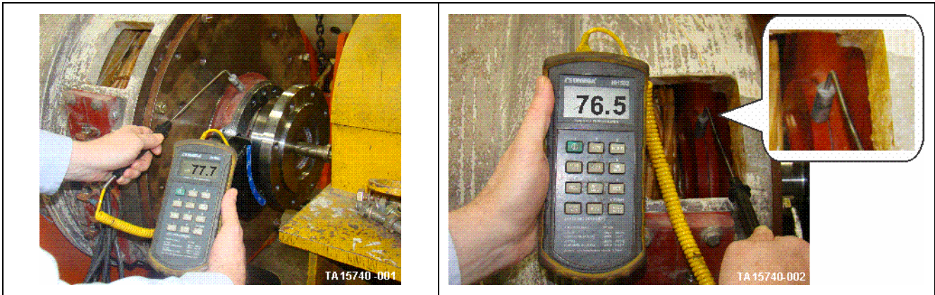
Figure 199. Typical temperature bearing testing
