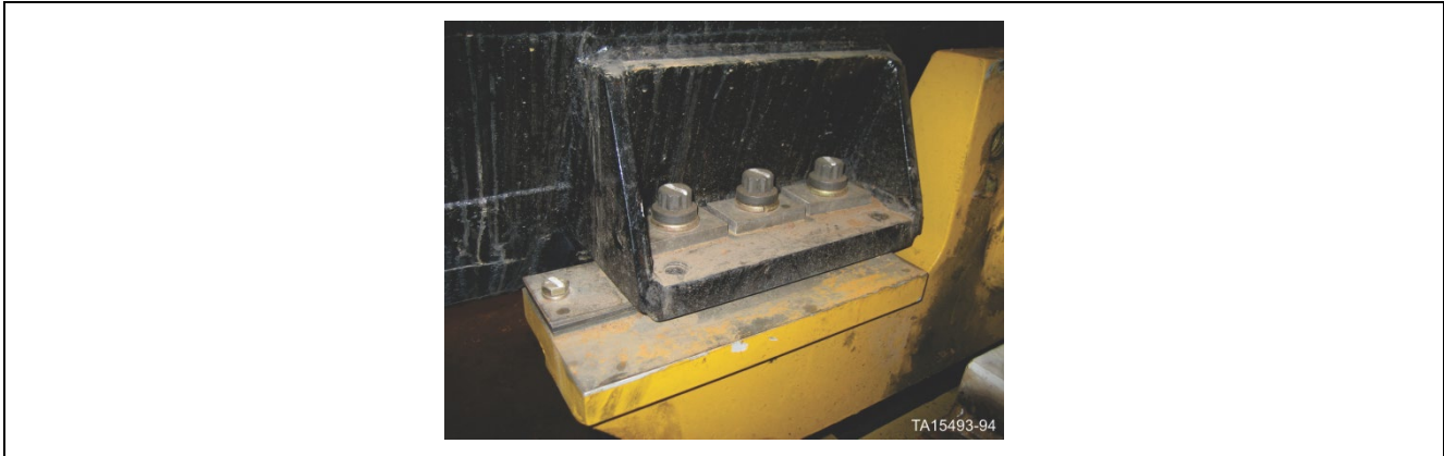
Figure 192. Shim pack installed at the generator mount foot
