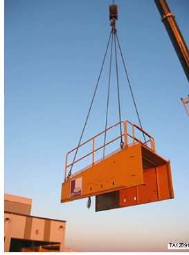
Figure 57. Hoisting the hood assembly
