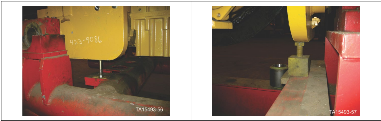
Figure 87. Support jacks under rear engine mount
