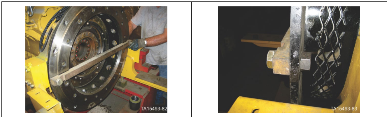
Figure 181. Straight edge installation
