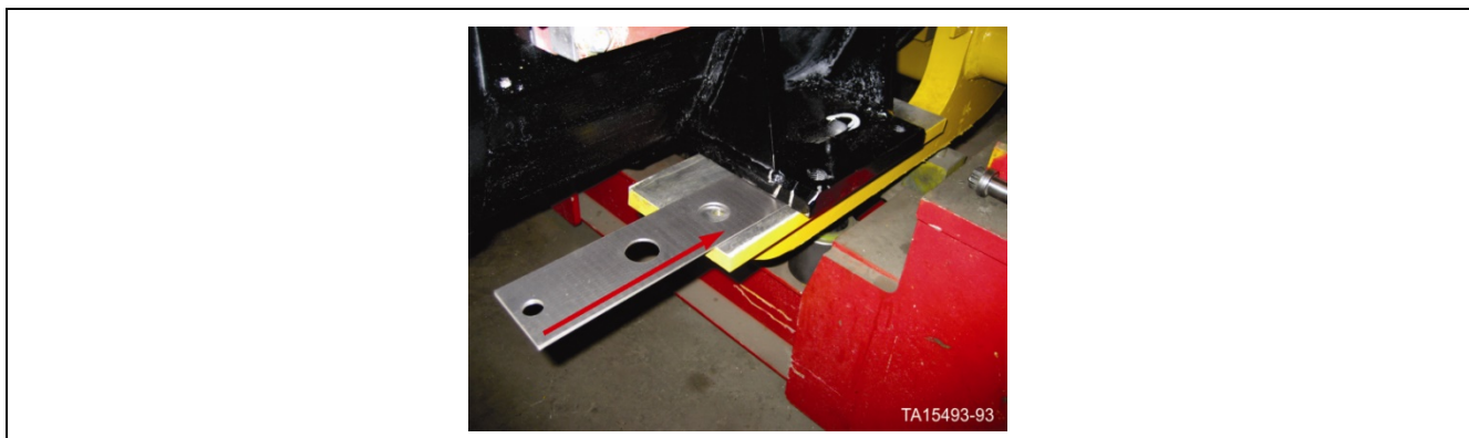
Figure 191. Installation of the shim pack at the generator mount foot
