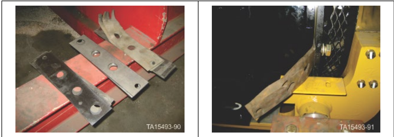
Figure 189. Install shims on both sides
