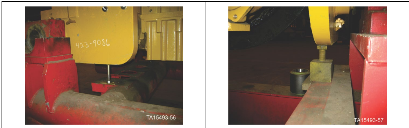
Figure 149. Jack bolt placed directly under the engine mount
